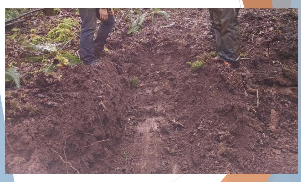
If this machine had been tethered, sliding and spinning of the tracks would not have occurred. The tether would have stabilized the machine on the hill
