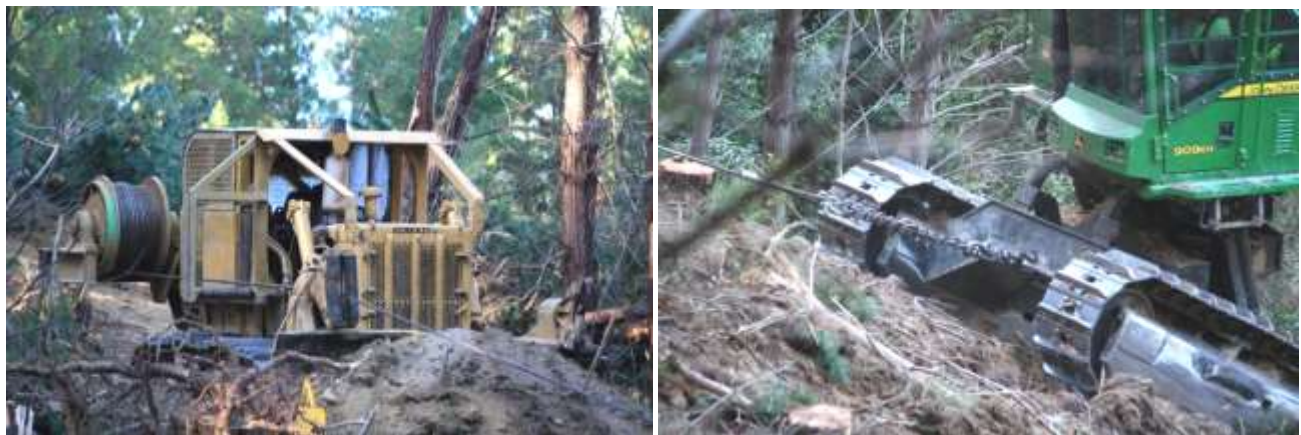
Figure 3: Purpose built self-levelling harvester (right) being cable assisted by the winch mounted on the dozer (left)
